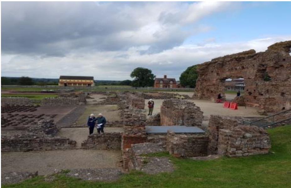
Picture 1 – an overview of the site
